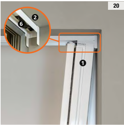
Align the box bracket with the cap.
